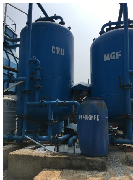
Filter Units for Color Removal and Suspended Solids
