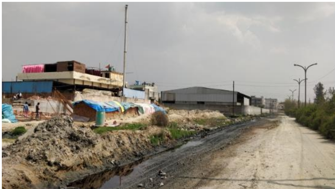
Wastewater in Industrial Estate
