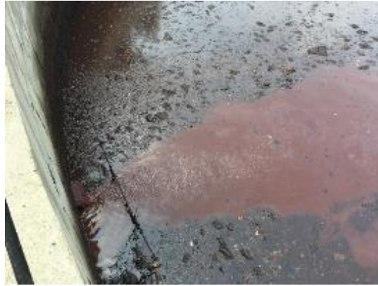
Inlet Equalization Tank
