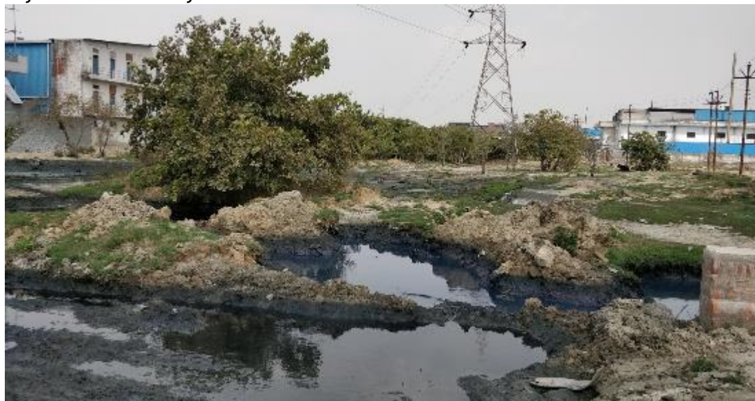
Wastewater outside CETP
