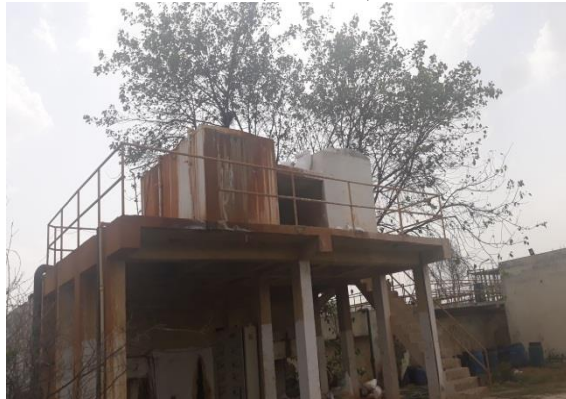
Lime milk & FeSO 4 preparation Tanks
