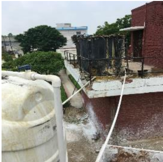
Chemical Storage for Flocculation
