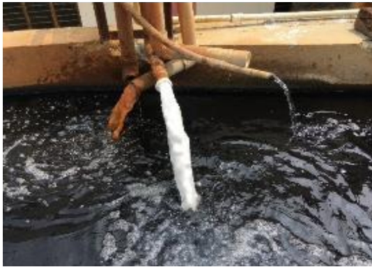
Current Primary Flocculation
