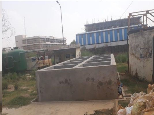
Sludge Drying Beds ( Construction under progress )
