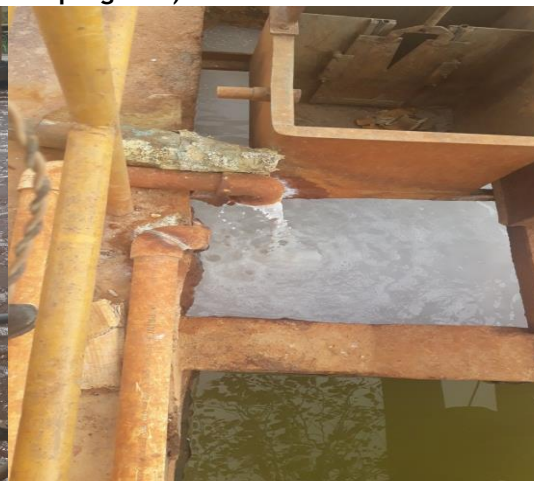
Segregated Lime & FeSO 4 Dosing in Physico-Chemical Treatment Section of CETP
