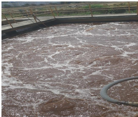
A View of aeration Tank with Leakages from Air Diffusers
